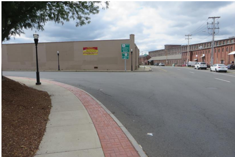
An extremely wide turning radius for motor vehicles and the lack of a marked crosswalk present safety challenges for pedestrians at the intersection of Front Street and Cabot Street.
