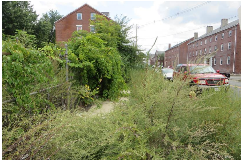
Overgrown sidewalks on Dwight Street should be cleared to ensure safe pedestrian access.
