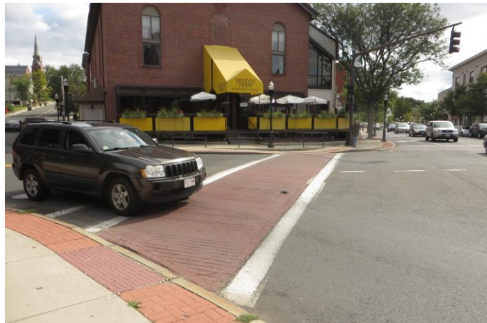
Wide turning radii for motor vehicles present safety challenges for pedestrians at the intersection of Exchange Street, Center Street and Springfield Street.
