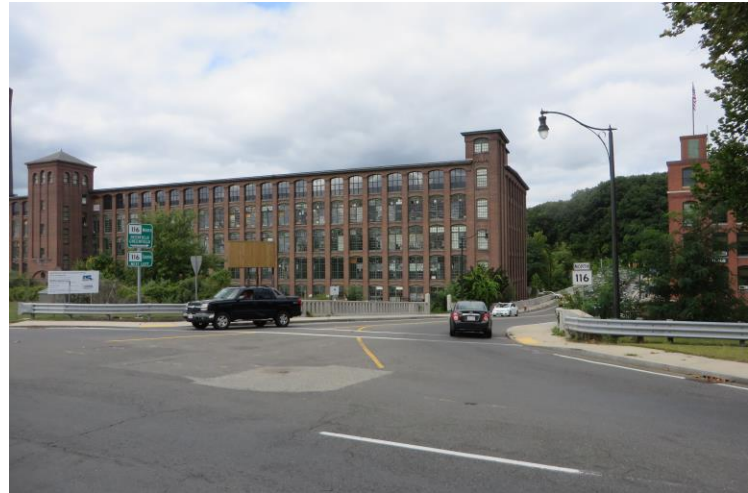
Long crossing distances and wide turning radii for motor vehicles present safety challenges for pedestrians at the intersection of Front Street and Springfield Street.
