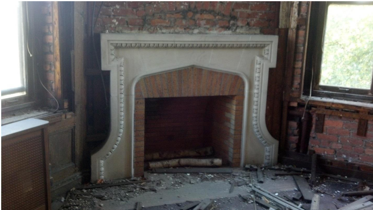
Building #26 – Original office fireplace
