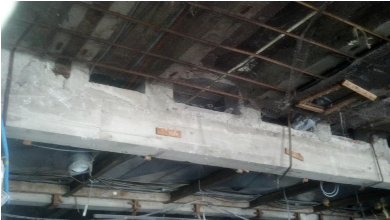
Building #26 – Interior abatement progress
