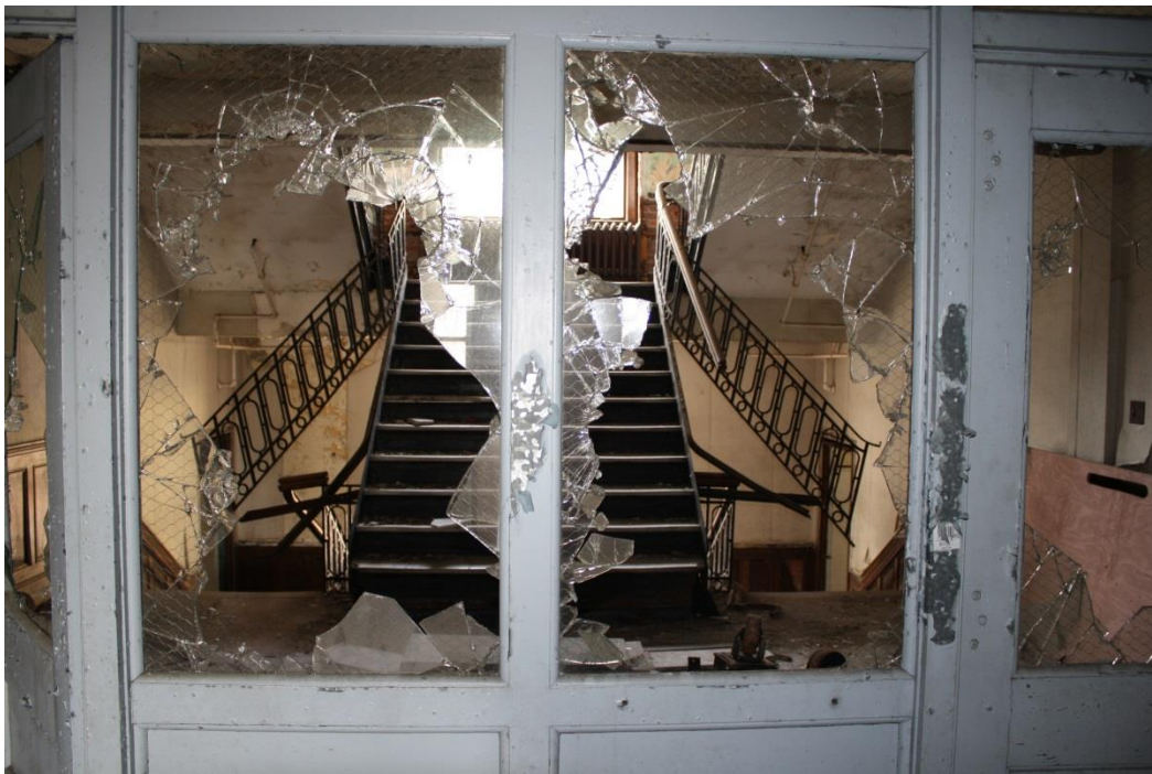
Building #26 – Central Staircase prior to abatement activities
