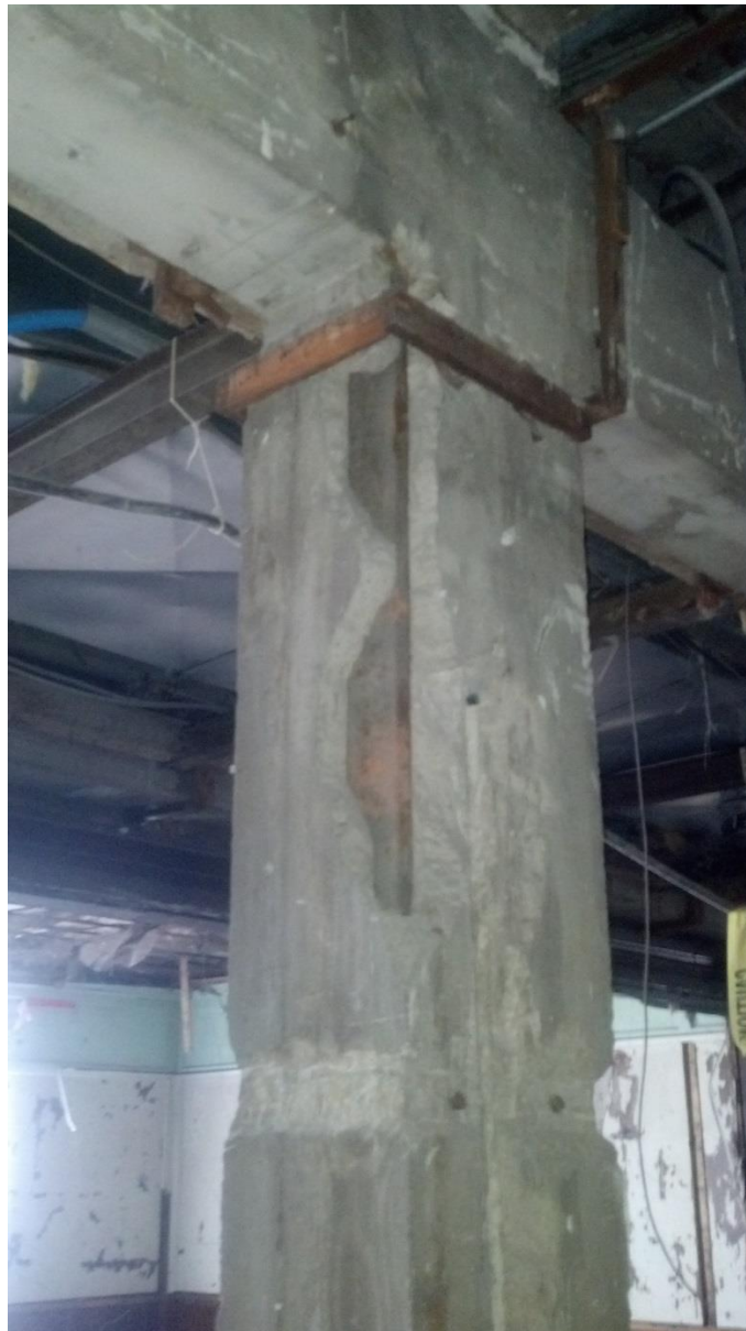
Building #26 – Removal of building materials from concrete columns
