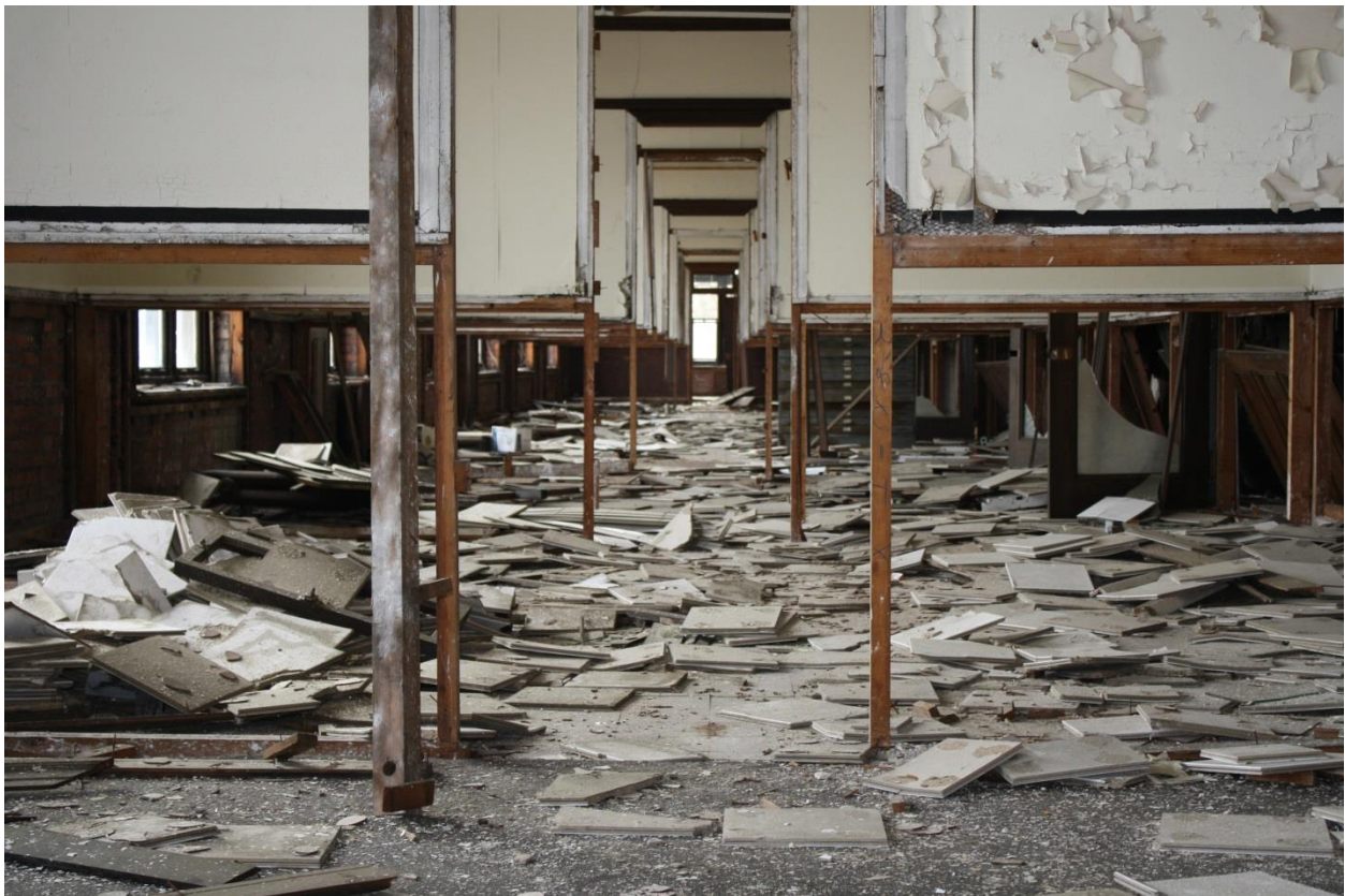
Building #26 – Interior of office floor prior to abatement activities
